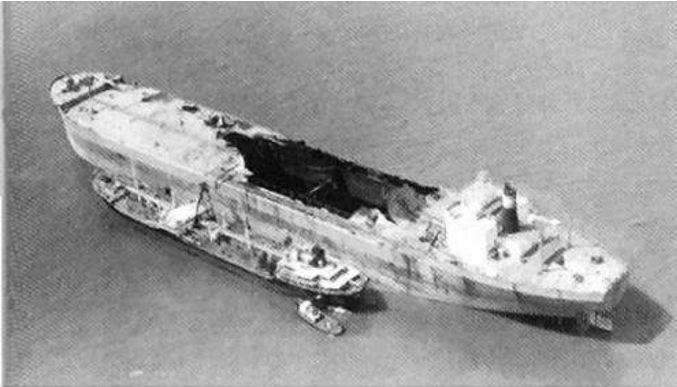
Figure 3: Kong Haakon deck after tank cleaning explosion. Obvious similarity to Mactra. Source: Auke Visser, supertankers.topcities.com
