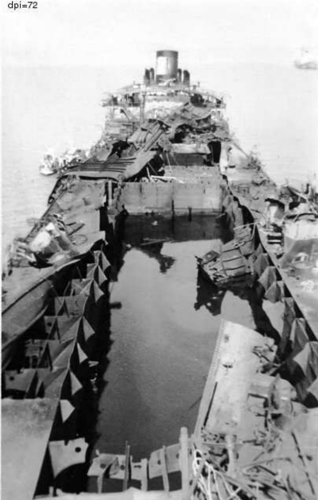
Figure 1: Stanvac Japan after tank cleaning explosion. 19 killed. Source: Ships Nostalgia
