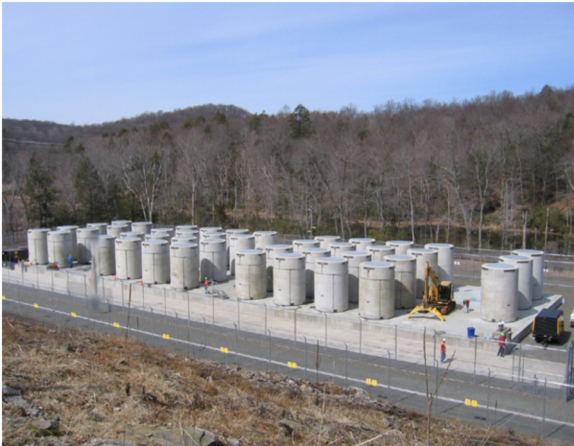
Figure 1: Connecticut Yankee Dry Storage Facility
